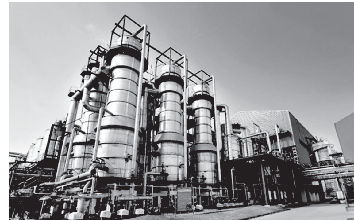
A view of the sugar refinery and cogeneration power plant set up at Sugar Unit-Hariawan in 2018.
